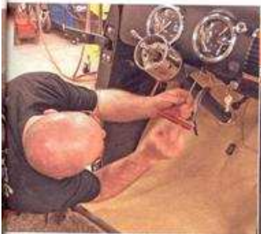
The steering column goes in, enabling the interior wiring to be completed.
