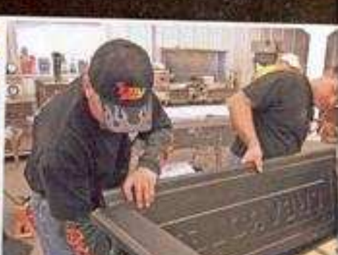
The tailgate is installed to finish the sheetmetal on the truck; care was taken to fit the panels perfectly.
