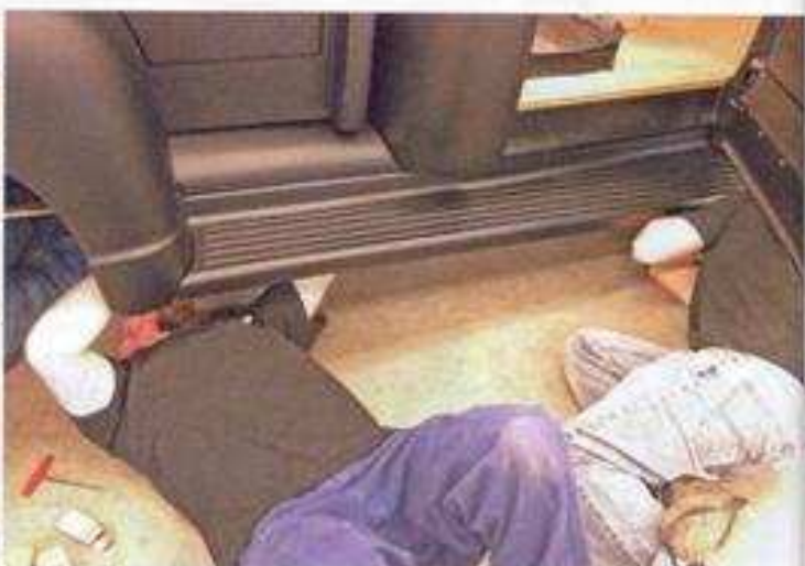
Two other team members are busy installing the running boards.
